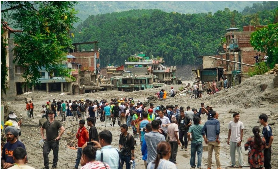
Project HOPE's team in Nepal surveys damage in Devighatz, where flash floods caused widespread destruction and buried entire stories of buildings under a thick layer of mud. Photo by Sandesh Tamang for Project HOPE, 2026.
